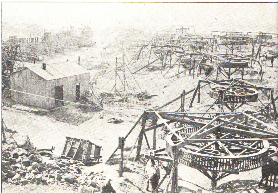
The platforms at the mine's edge had three levels – the top for cables going to the centre of the crater, the middle and the bottom for cables progressively closer to the precipitous sides of the gaping, man-made crater.
