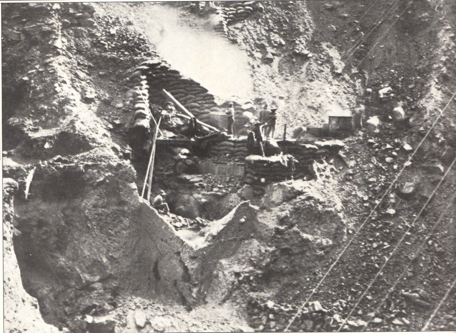
Mining at the edge of the crater was plagued by persistent rock falls and diggers were for ever reinforcing the sides of their claims with sandbags.
