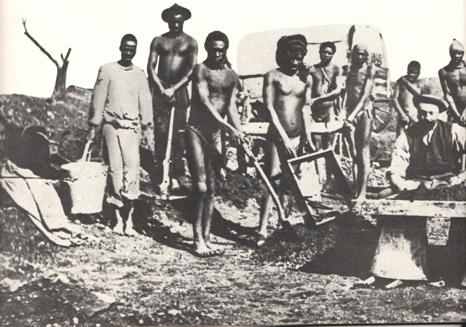
After sieving the diamond-bearing soil, many diggers washed the material in hand-rotated drums to reveal the elusive stones.
